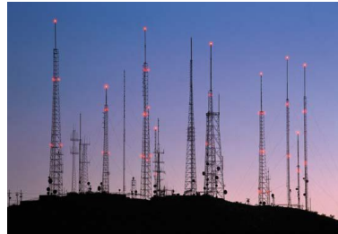
Antenna array system
